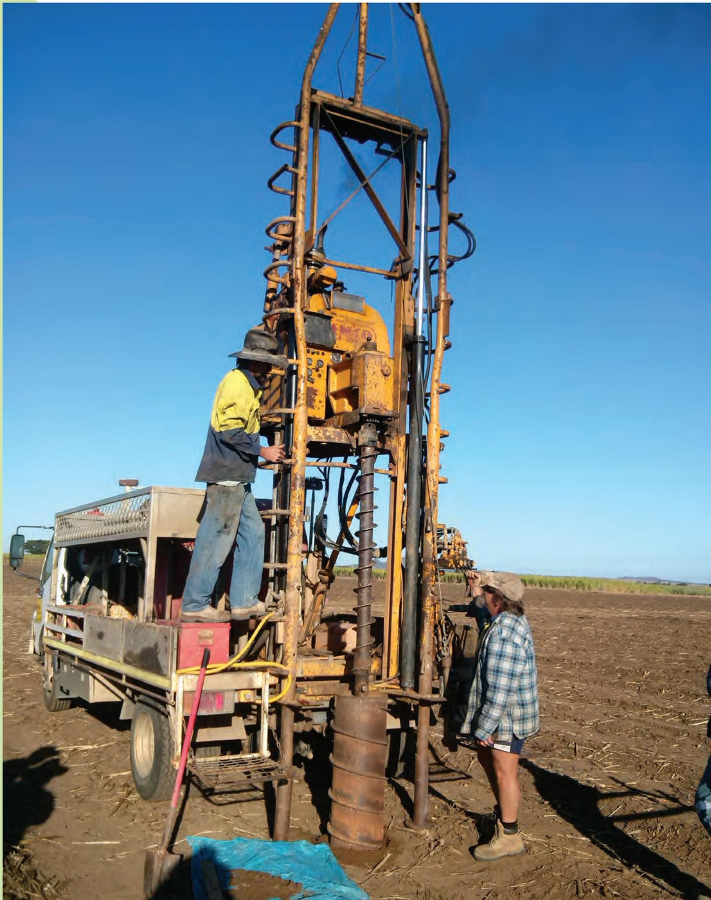
Above: Drilling cores for lysimeter installation at Ayr Farming, Project Catalyst trial site.
