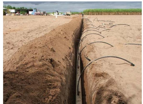
Underground pipes connect all the rows of irrigation equipment together
